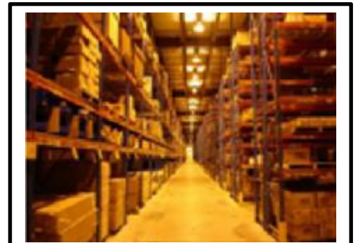
THE VISUAL PERCEPTION PROBLEM: A warehouse illuminated with HPSV lighting
