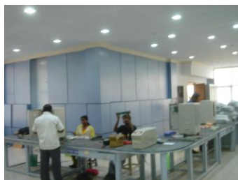
All factory illumination is with our 12W LED Downlighters. About 80 Downlighters have been used over a 5500 sq. feet area to achieve a lux level of 250 Lux on the work plane, as this is going to be an electronics factory.
