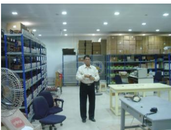
All factory illumination is with our 12W LED Downlighters. About 80 Downlighters have been used over a 5500 sq. feet area to achieve a lux level of 250 Lux on the work plane, as this is going to be an electronics factory.
