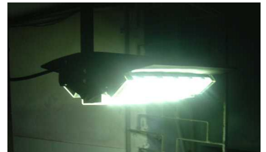
BINAY's 'Eagle-Eye' LED Pendant High Bay Luminaire has an arrangement for adjusting the beam pattern, which allows wide angle dispersion of light
